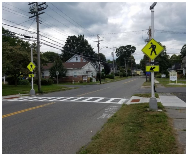
Figure 6.2: Crosswalks with Rectangular Rapid Flash Beacon (Photo Credit City of Poughkeepsie, NY)
