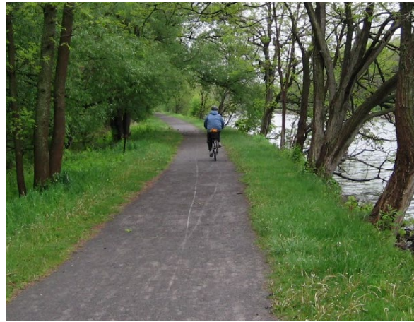
Figure 7.1: Multi-use Path with Stone Dust Surface
